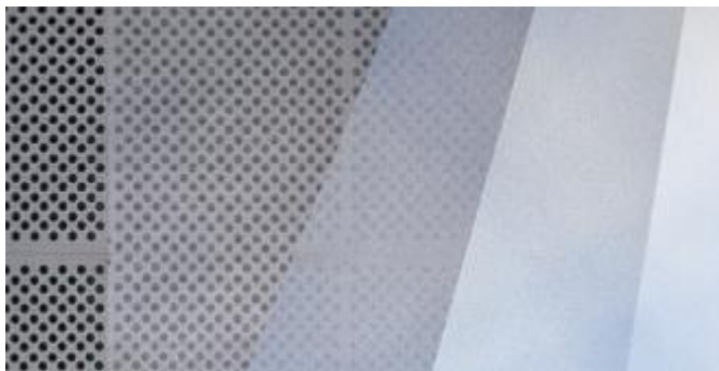
Layer build-up of the finishing coats
